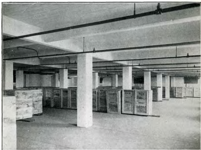
Interior of No. 1 Store House. Note perfect condition of building and contents.
