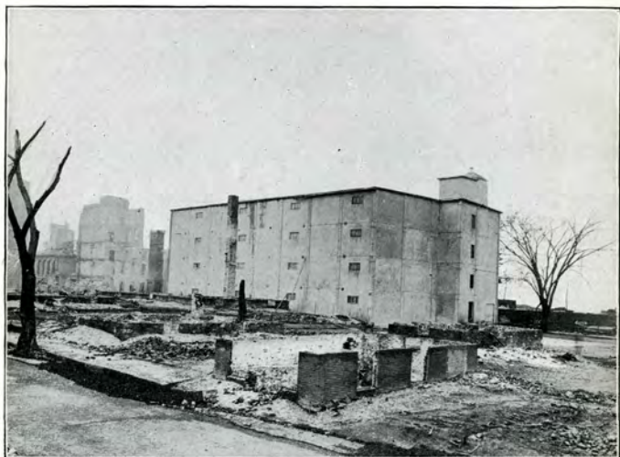
No. 1 Store House. Reinforced concrete construction. Practically uninjured though severely exposed.
