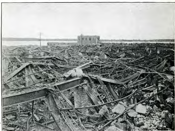
Wreckage. Floor beams, etc., No. 6 Weave Building.
