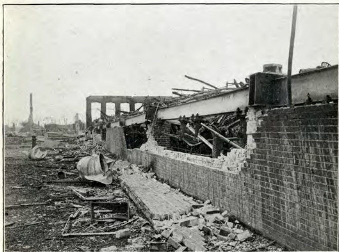
South Wall, No. 6 Weave Building, thrown over by expansion of steel floor beams.
