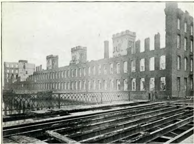
North Side of No. 2 Mill. Burned bridge in foreground.
