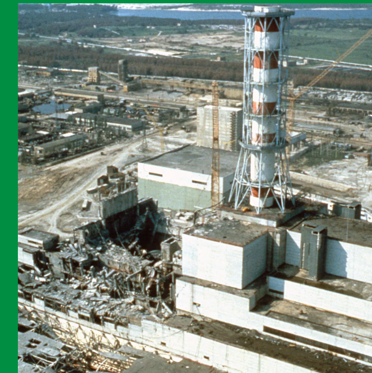
Figure 1. The aftermath of the reactor meltdown (Walker, 2020).
