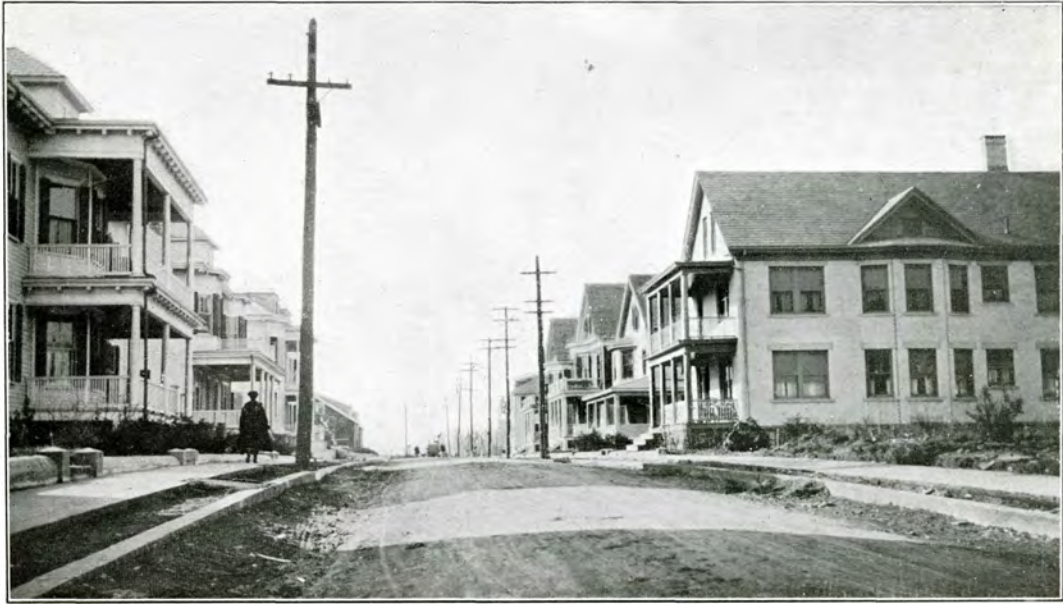
HOLLY STREET All new houses, but no trees
