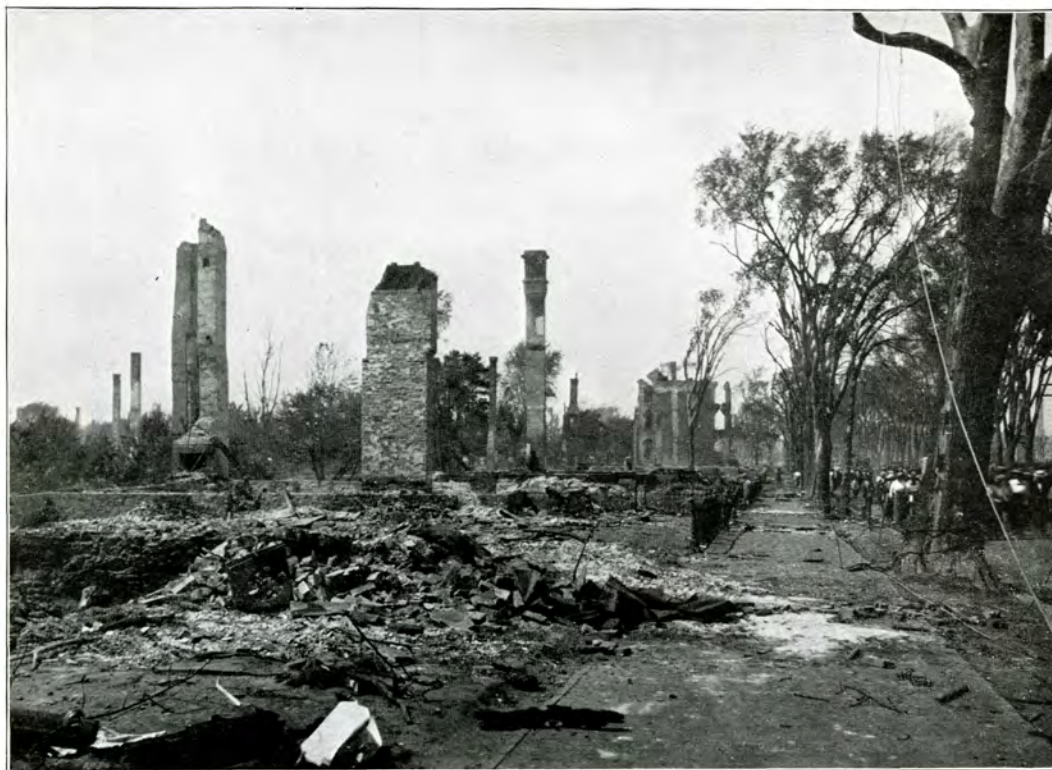
LAFAYETTE STREET Immediately after the fire of June 25, 1914. All trees in the picture were killed
