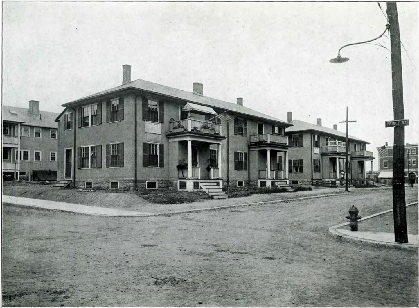
TYPE OF FOUR FAMILY HOUSES BUILT BY THE NAUMKEAG STEAM COTTON CO.
