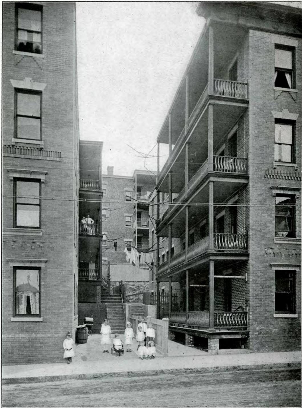
PLENTY OF LIGHT, AIR AND HEALTHY CHILDREN BETWEEN 52 AND 56 WARD STREET Compare with picture on opposite page of types of construction before the fire. Both pictures were taken in the "Point" district.
